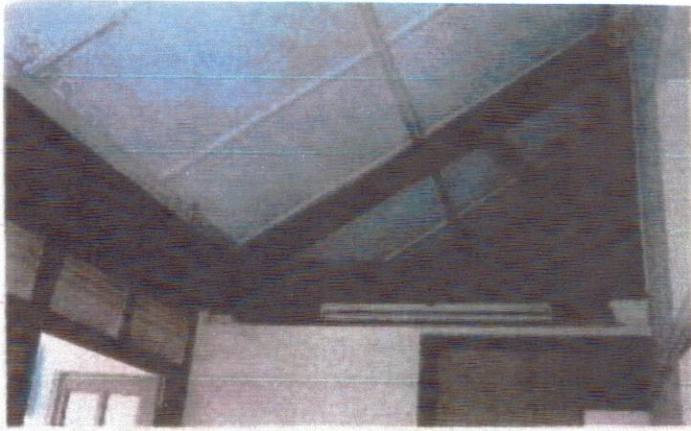
DETAIL OF EXPOSED TRUSS AT BALCONY
