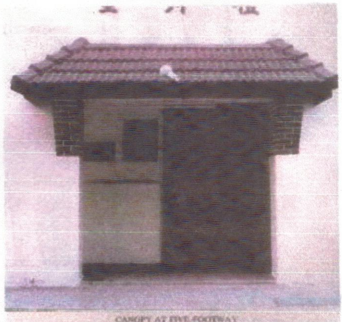
CANOPY AT FIVE-FOOTWAY
