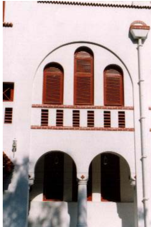
Arc timber window with cast iron water downpipe
